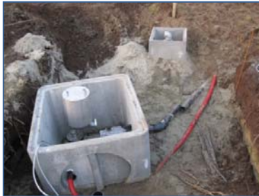
Figure 4: View of injection filter equipment and manhole cover in construction
