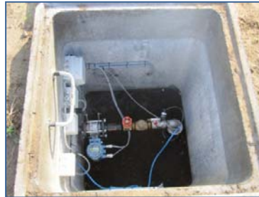
Figure 5: View of extraction filter equipment and manhole cover finished
